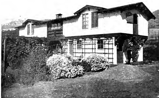
BARN AND PUMP HOUSE OF DUNCAN McDUFFIE, ESQ., BERKELEY, CALIFORNIA John Galen Howard, Architect
